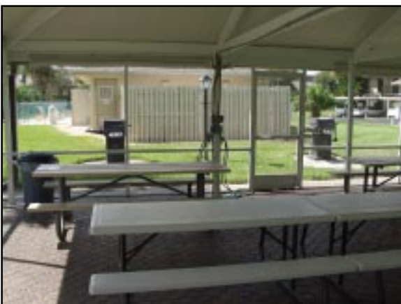
Inside Tables, Lighting, and Ceiling Fans
